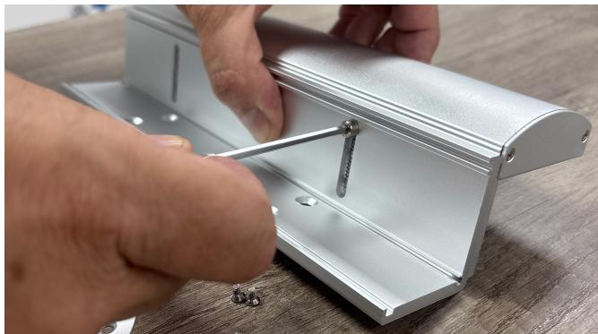
Secure the two sections of the Z-bracket (**A** & **B**) using the four screws (**D**).
