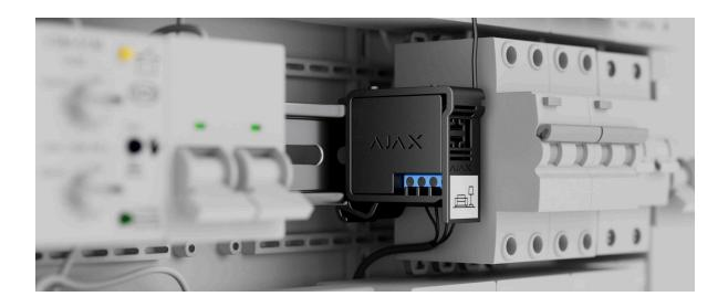
A 39 × 33 × 18 mm device is connected to the circuit gap. Relay Jeweller dimensions allow installing the device into the deep junction box, inside the electrical appliance enclosure, or in the distribution board. A flexible external antenna ensures stable communication. To install Relay Jeweller on a DIN rail, we recommend using a **DIN Holder**.
